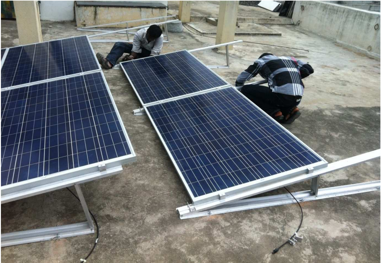
Fig 9.0 Installation of Solar system at Vellore – 2 kWp (Off Grid)
